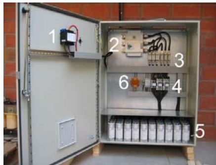
Figure 7: Condenser battery (source: Wikipedia) '5' being the capacitors
